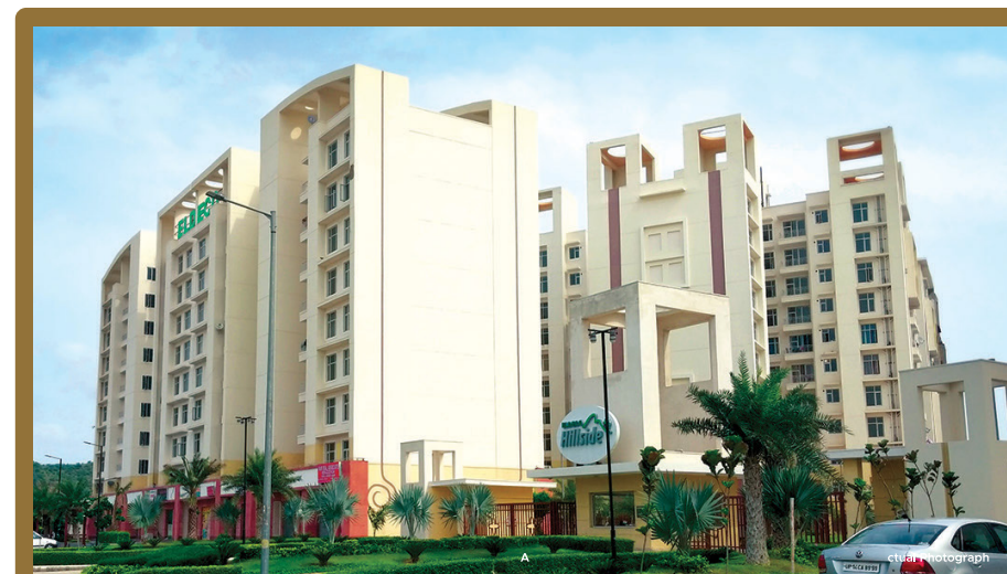
Eldeco Hillside, Japanese Zone, Neemrana
